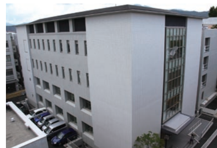
iCeMS Research Building: Located at the "Hyakumanben" intersection, about 200 meters from the iCeMS Main Building
